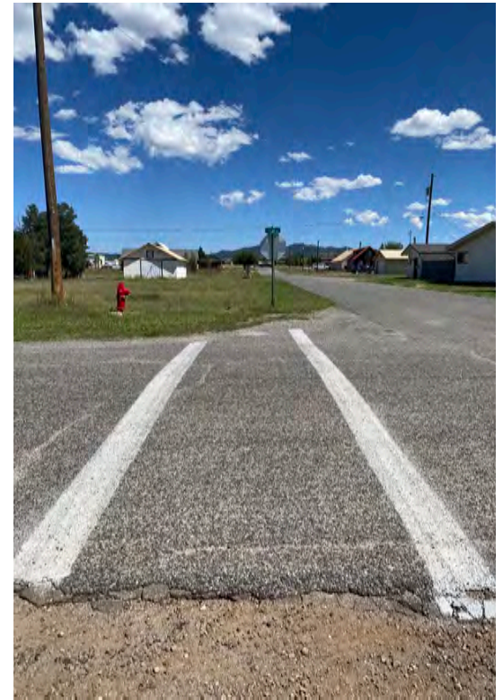
Existing crossing by Memorial Park.
