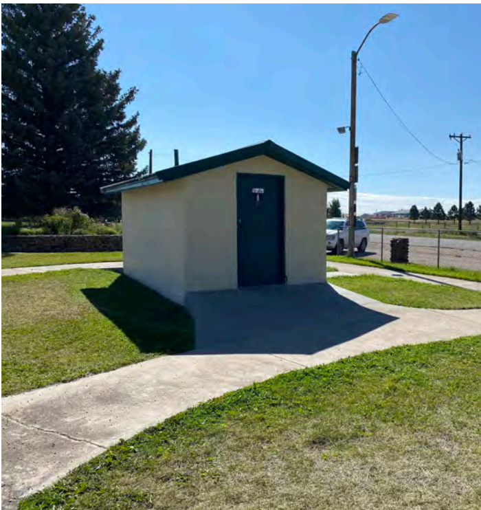
Existing bathroom at Memorial Park
