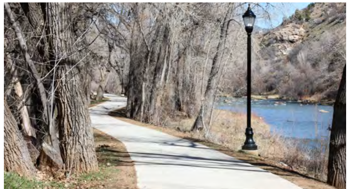
Example of a Concrete Paved trail.
